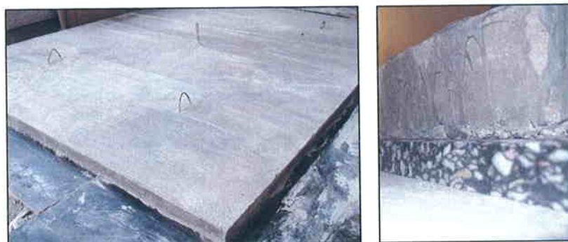
Images 8 and 9 – Concrete slab and its installation over Recfoam ® U150 panel
