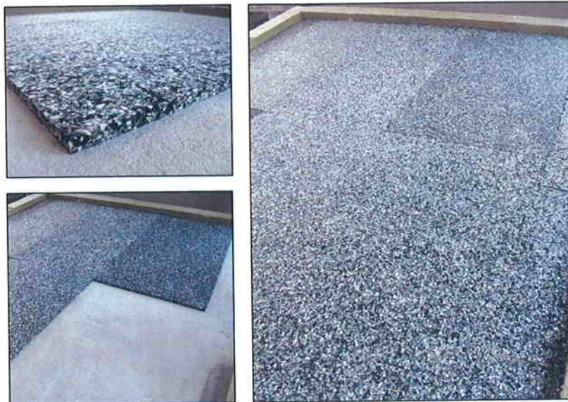
Images 5, 6 and 7 - The panel is placed over the basic concrete floor
